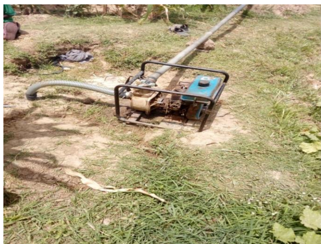
Figure 2: Water pumping Machine use at shallow water table 10-12m dept
